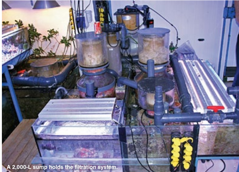
A 2,000-L sump holds the filtration system.
